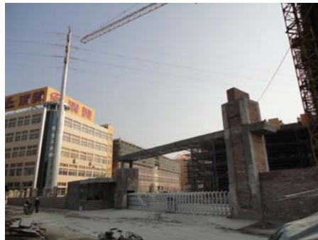
R&D Centre under construction
