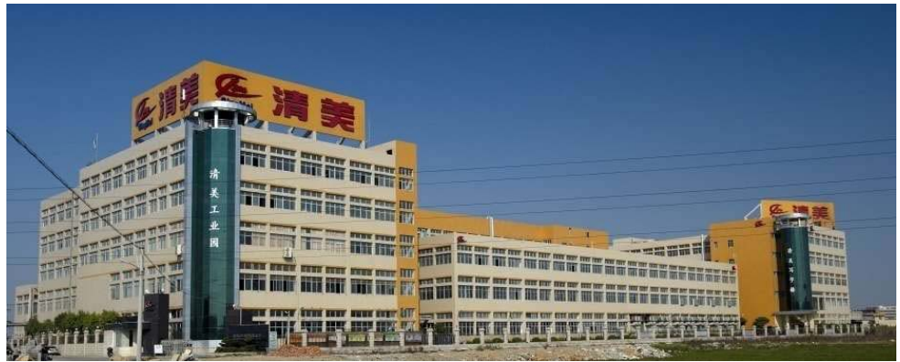
Old Production Facility
